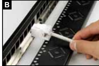
Position the shielded keystone jack for installation.
